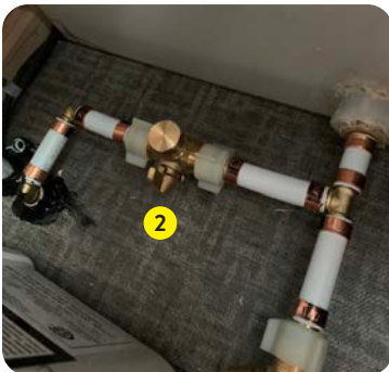
2. Drinking water drain valve
